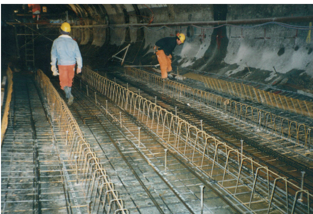
BKW Tunnel Tunnel BKW
